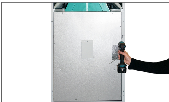
3. Remove the screws and demount the cover plate.
