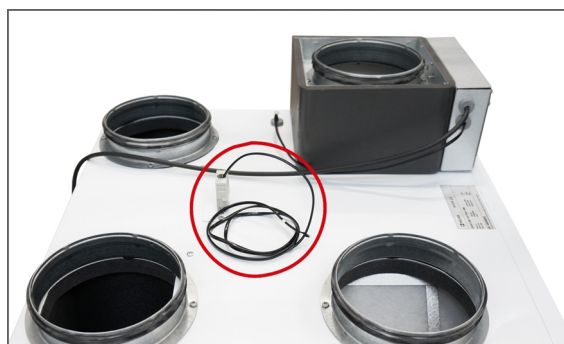
6. The T1 sensor is pulled from the 8-pole outlet into the outdoor air duct (30 cm before the preheating surface).
